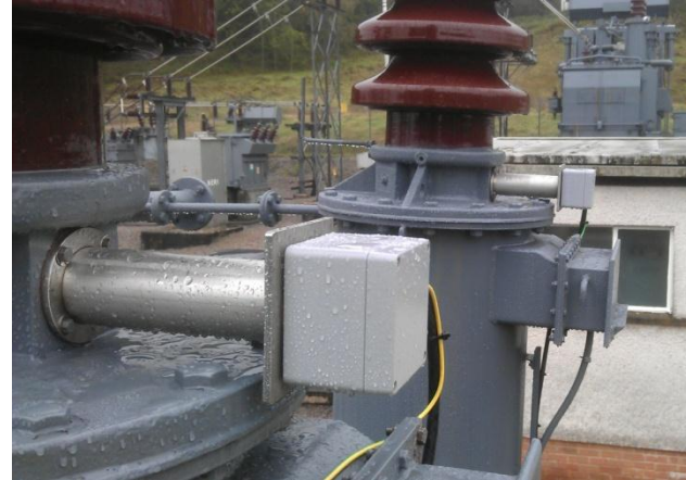
132KV / 300A Bushing from Brush
