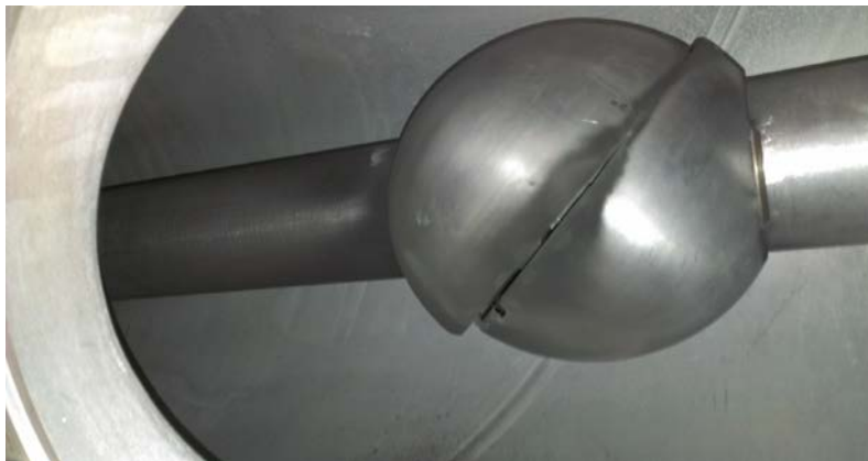
Stress Cone Fault (2012)
